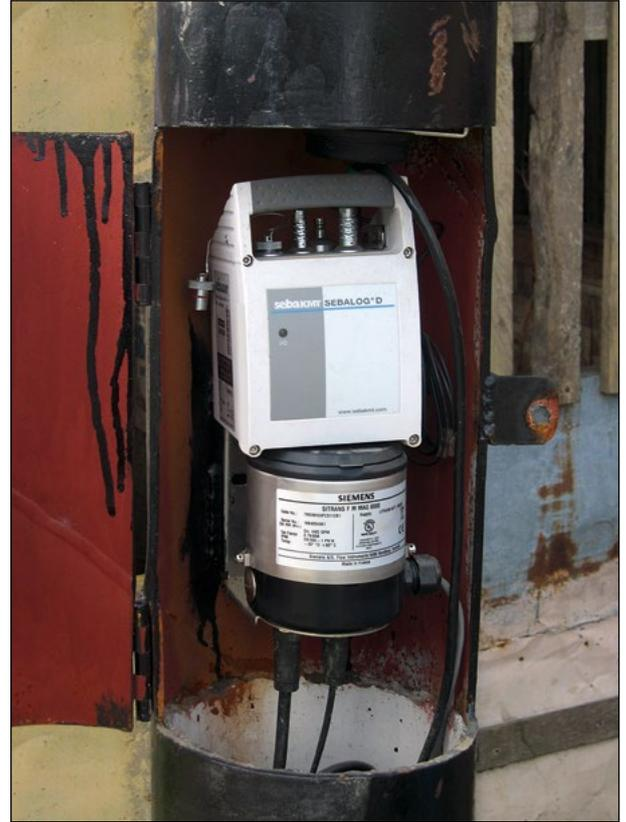
Sebalog Dx data logger connected to a flow meter
